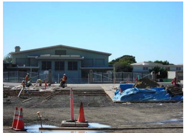
Main Courtyard: Concrete Walkways & Fence
