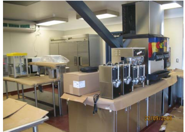
Concession countertops and equipment
