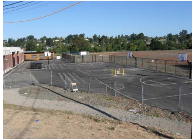
Installation of (N) Basketball Courts-COMPLETED
