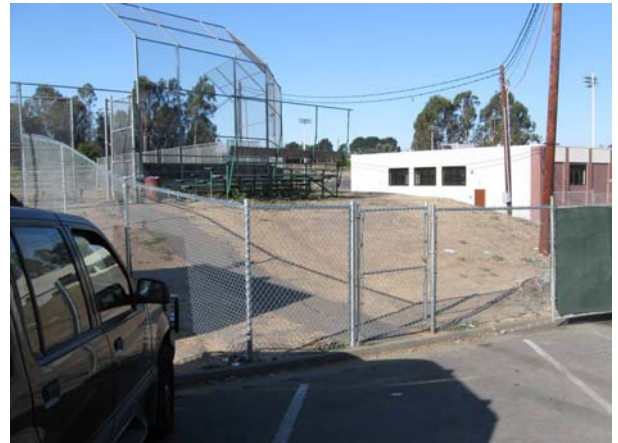
Installation (N) Site Access Fence-COMPLETED
