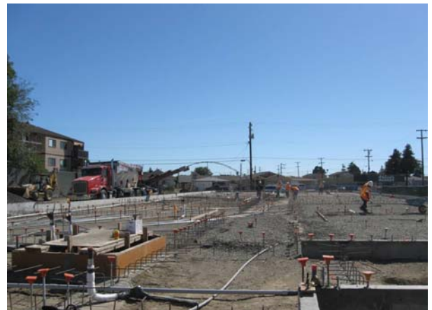
Placement of Rock in Building Pad
