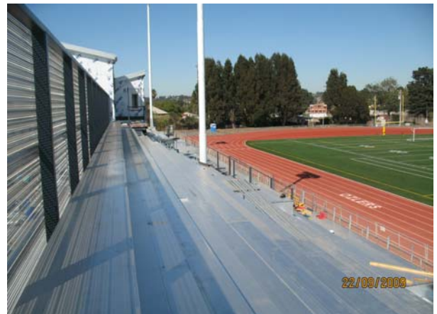
Bleacher planking installed and ready for seating
