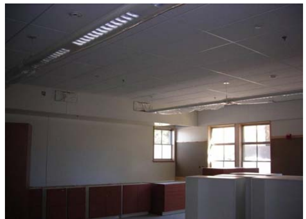
Bldg C1: Interior Finishes & Teaching Walls
