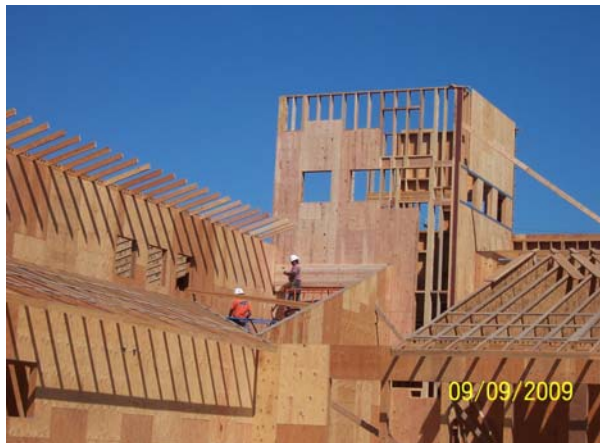
Building A West - Roof and Tower Framing
