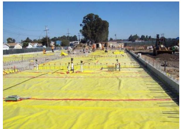
Installation of Under-Slab Water-Proofing
