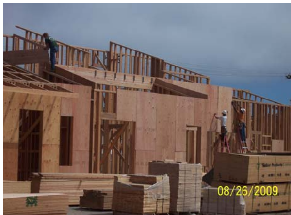
Building A East - Wall Shear Ply and Roof Framing
