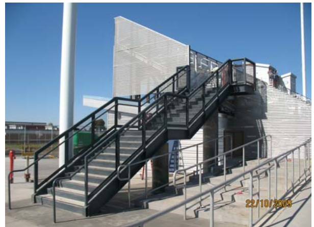
Main egress stairs poured and completed
