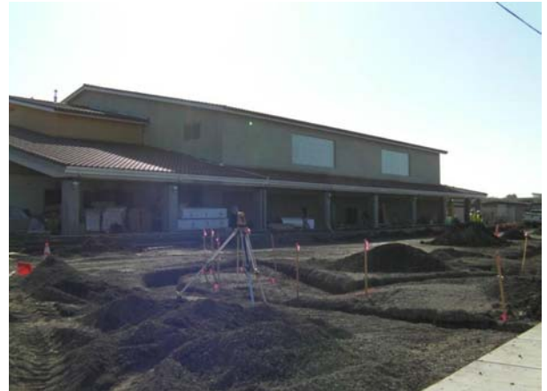
Visitor Parking Lot: Curbs poured & dug
