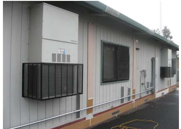
Installation (N) Protective Screens-COMPLETED
