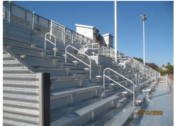
Bleacher seating, stairs and handrails complete
