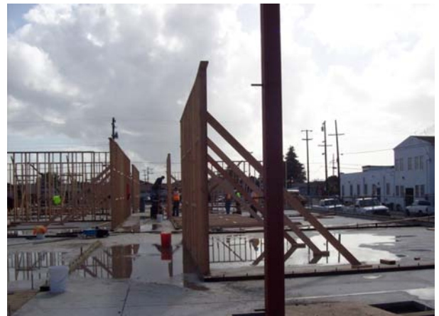
Construction of Interior Wall Framing at South End
