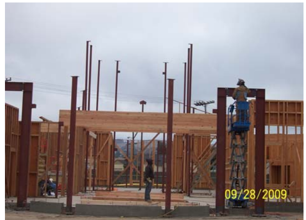
Welding of Steel Columns and Placement of GluLam Beams
