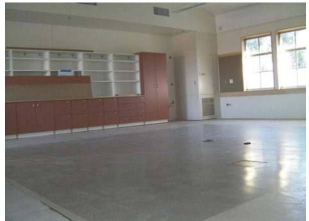
Bldg C1: Installation of VCT Flooring
