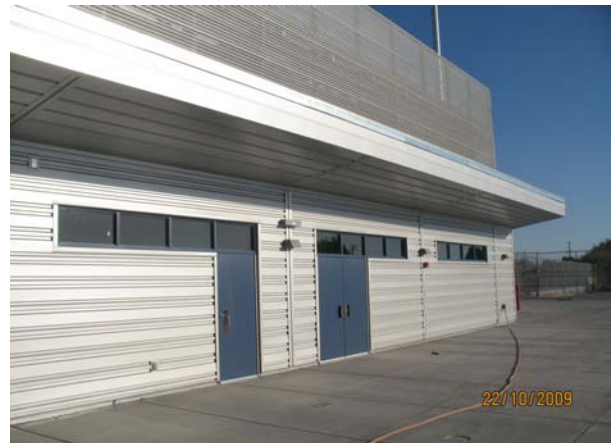
Completed exterior metal siding
