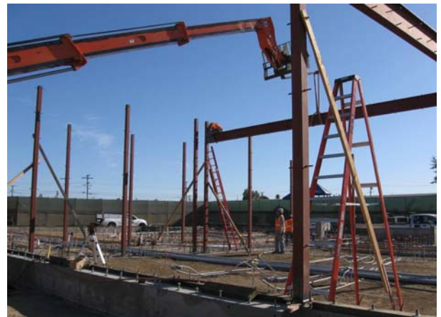
Erect Steel at North End
