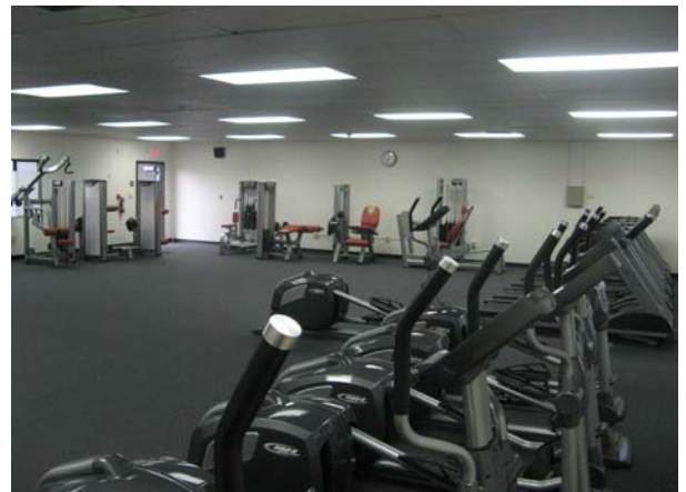
Installation of (N) Gym Equipment-COMPLETED
