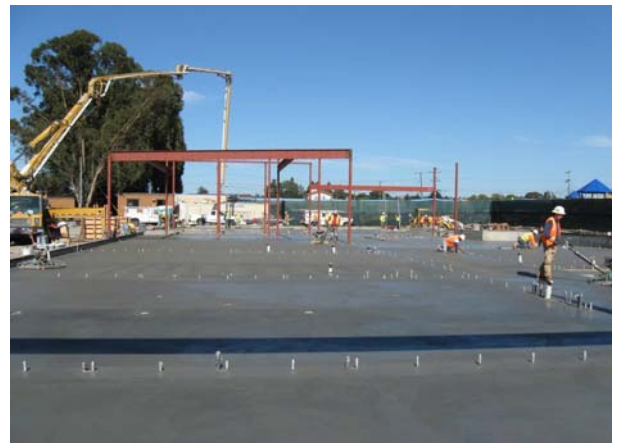
Placement of Concrete Slab on Grade
