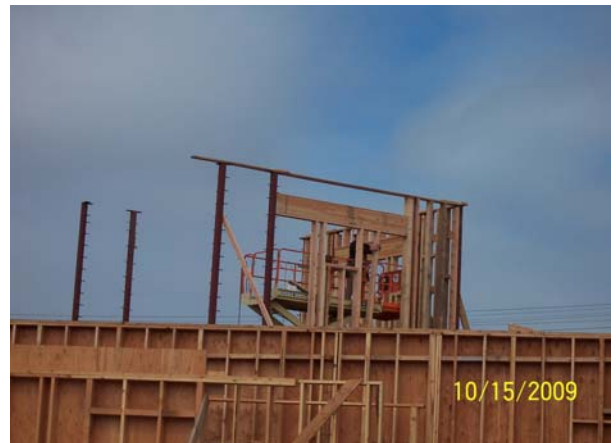
Tower Wall Framing and Shear Ply
