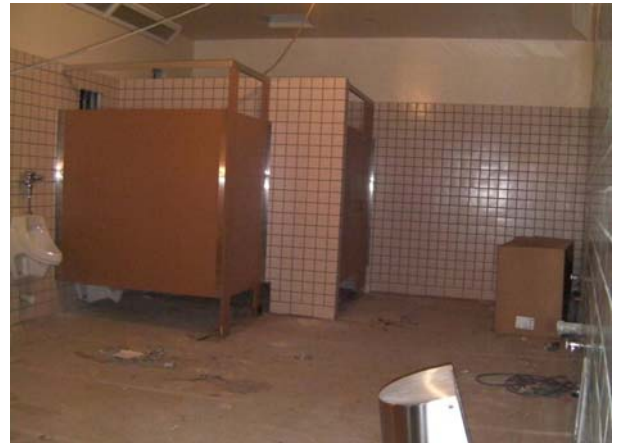
C Bldg- Boys Restroom: Partitions & Fixtures
