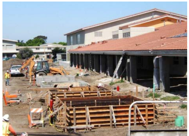
Main Courtyard: Planters & Roof of Bldg. MC
