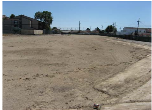
Increment 1A-Site Clean up and Demobilization-COMPLETED
