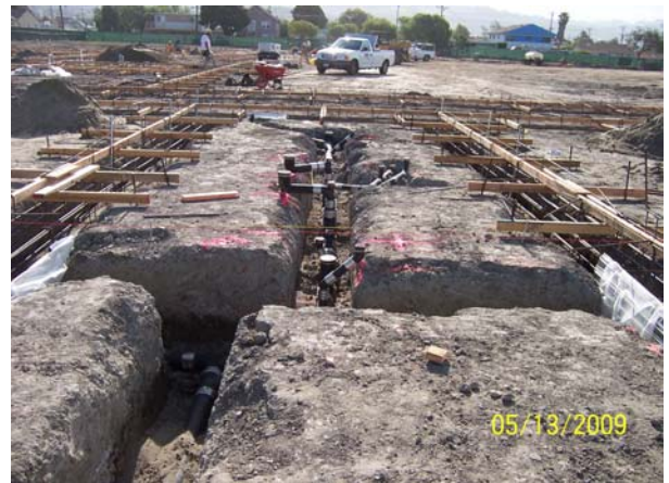
Underground waste and electrical rough-in
