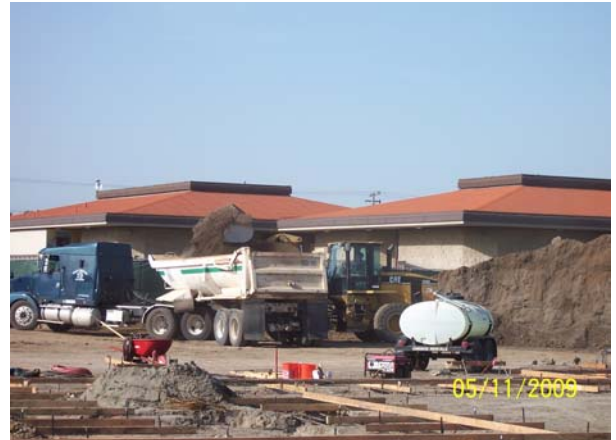
Off-haul of excavation spoils
