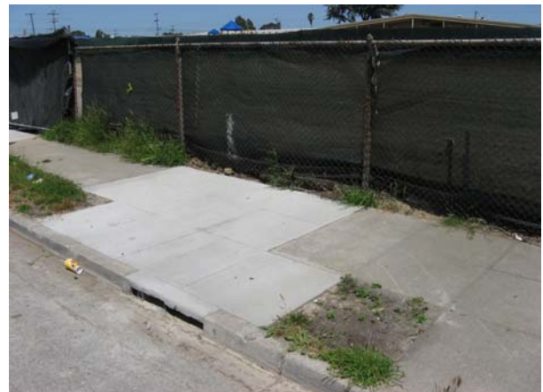
Increment 1A-Sidewalk Construction-19th Street-COMPLETED
