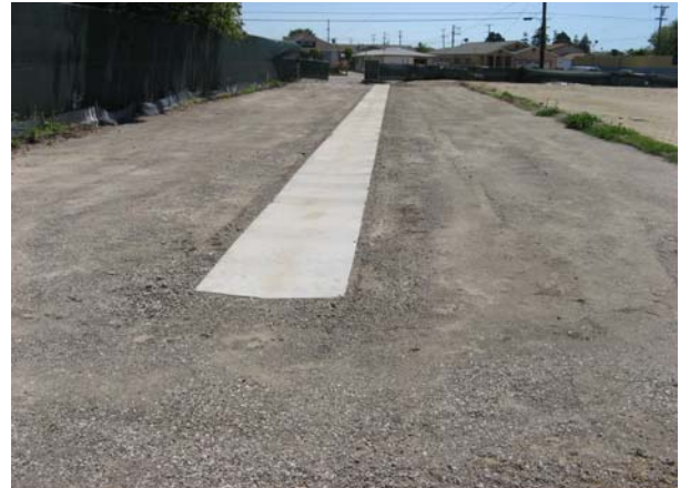
Increment 1A-Concrete Swale and Parking Area-COMPLETED
