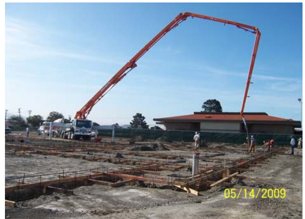
Concrete pour of footings at Building A west side
