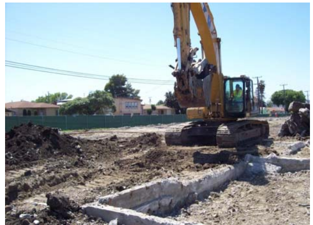
Foundation Removal Continuation
