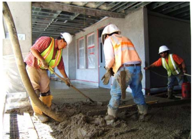
Building C: Installation of 2nd Fl. Topping Slab
