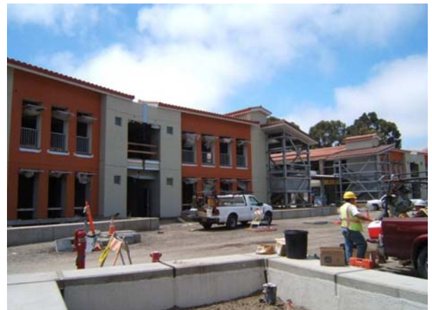
Main Courtyard view of C1 & C2 Locker areas
