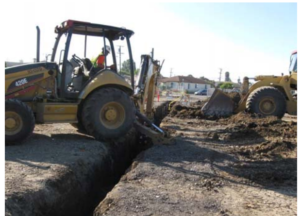
New Sanitary Sewer Installation
