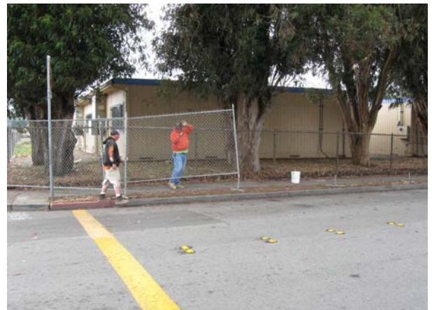
New Temporary Construction Fencing
