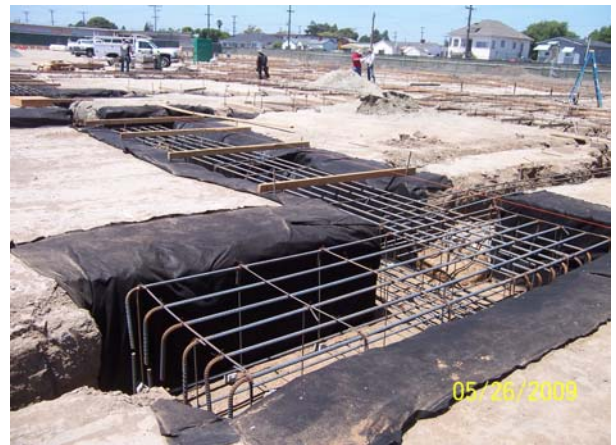
Rebar over filter fabric at footing brace frames
