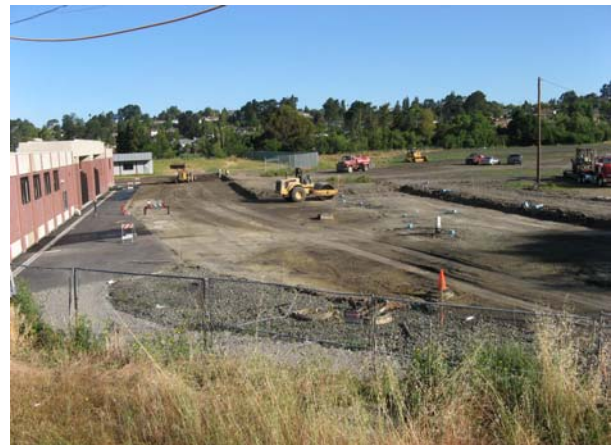
Excavation & Preparation for Base Rock-COMPLETED
