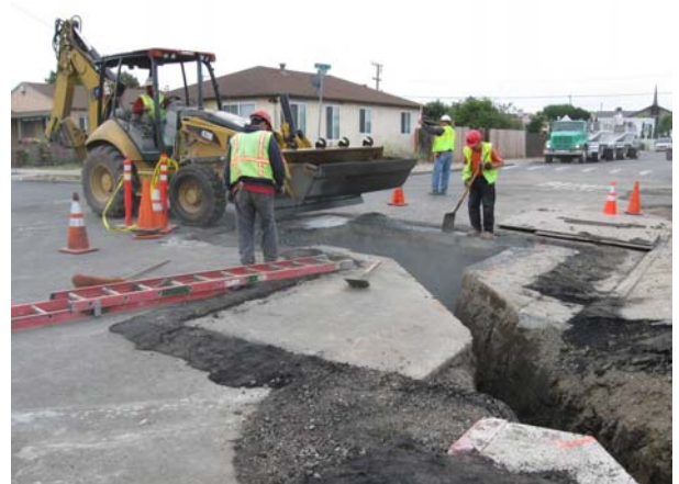
New Sanitary Sewer Manhole Installation
