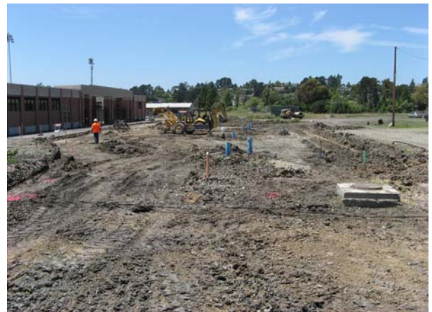
Removal of (E) Asphalt Paving & Site Prep-COMPLETED
