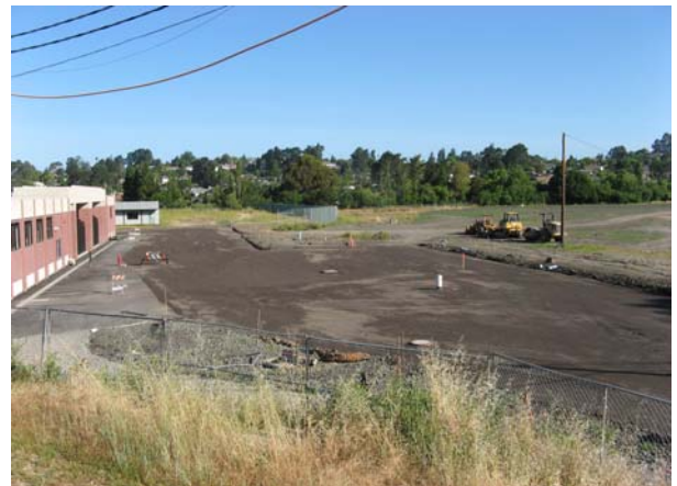
Base Rock Installed and Compacted-COMPLETED
