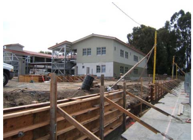
West Wall, Planters and Gates
