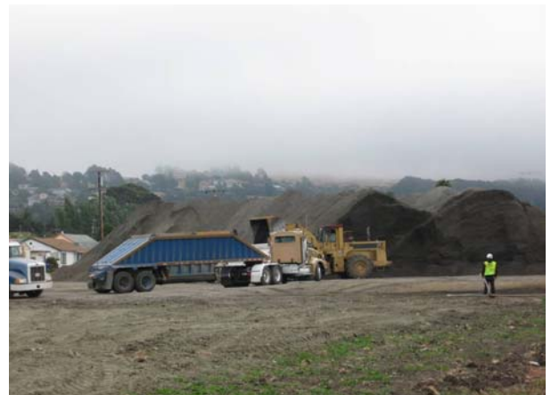
AC and Base Grinding Off-Haul
