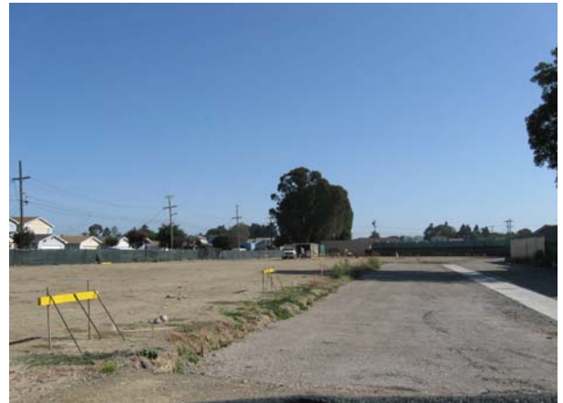
Building Pad Surveying & Staking
