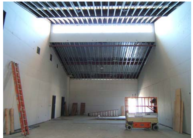
Building G: Interior Gyp & Clerestory Window
