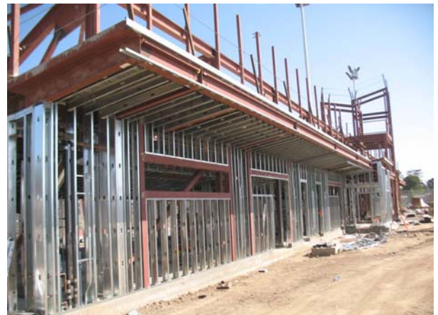
Exterior metal stud western facade framing
