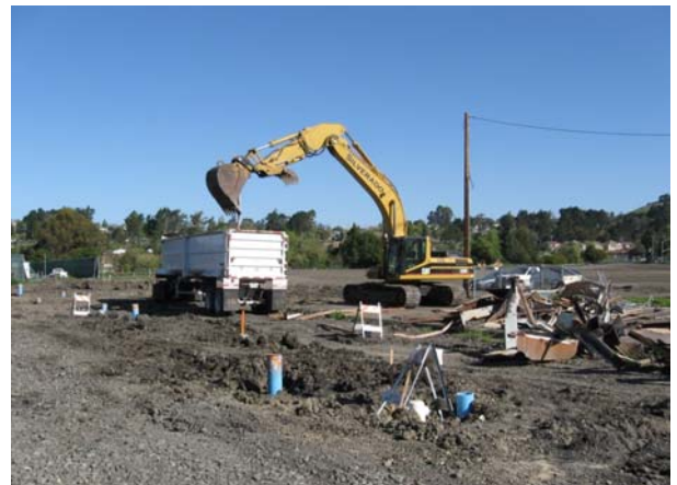
Temporary Portable Demolition
