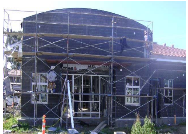
Building A: Windows, Storefront, & Lath
