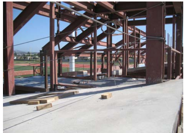
Concrete roof deck poured
