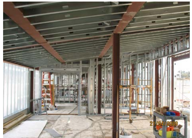
Interior wall and ceiling framing
