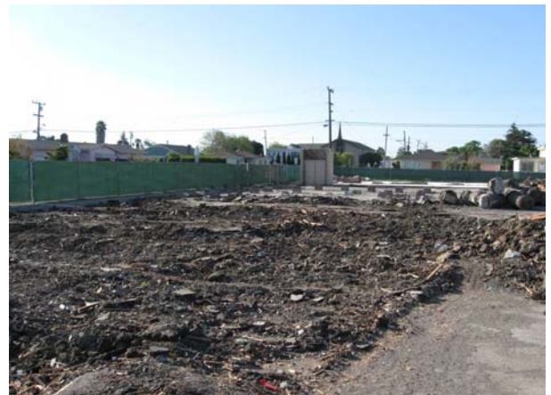
Footing and Foundation Removal
