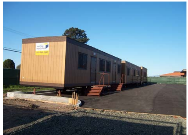
Construction Trailer Delivery & Set-up
