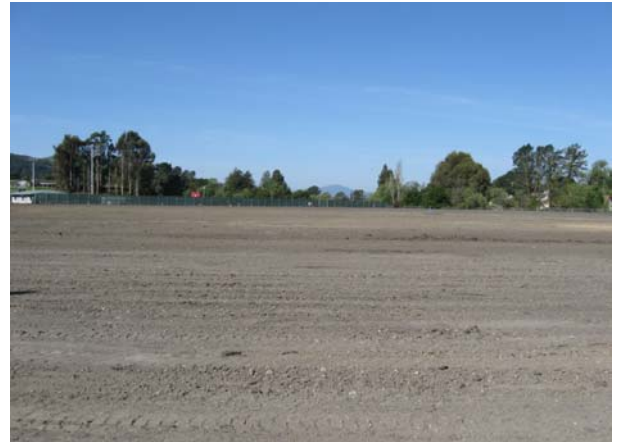
Fine Grading of Site
