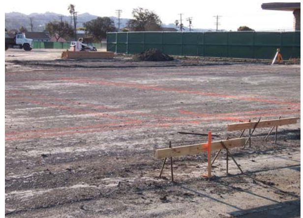
Site Survey and Footing Layout
