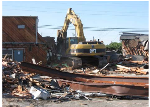
Existing Building Demolition
